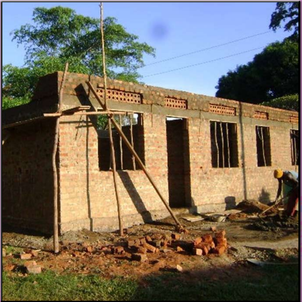
The Bishop's Guest house now at roofing stage
