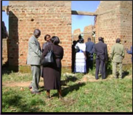
Part of Keyo Church under construction
