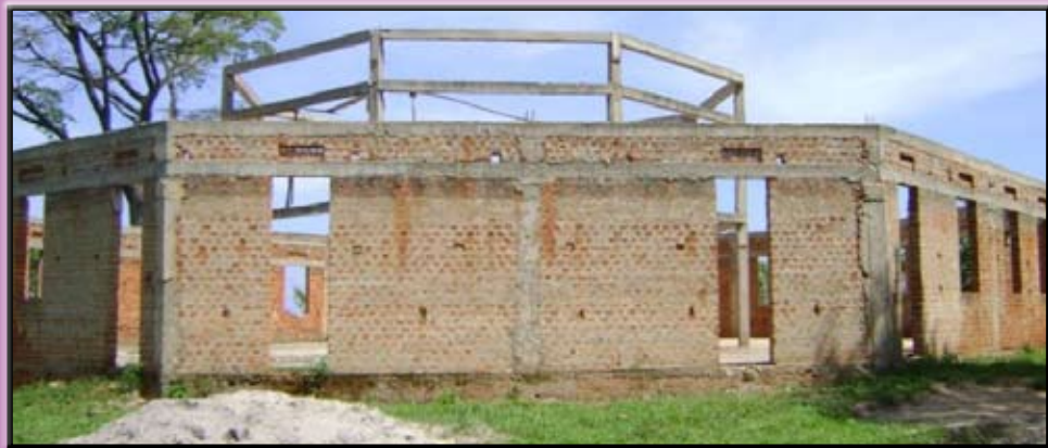
New St. Philip Cathedral under construction.
